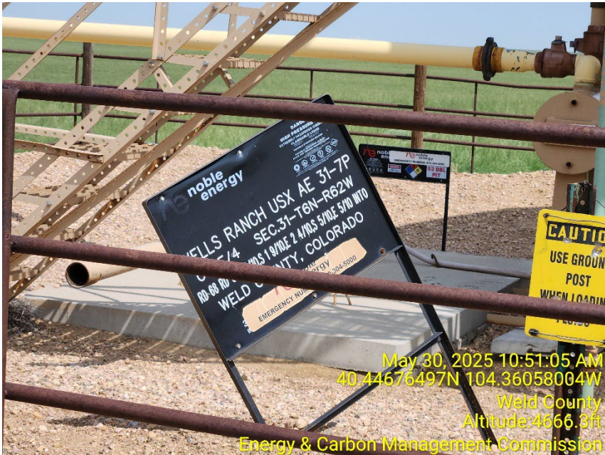
Photo 2 – Tank Battery Sign
