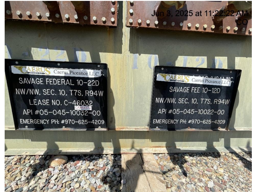
Photo # 5619 Emergency phone # on wellhead signs disconnected & not in service/not in compliance with CECMC rules
