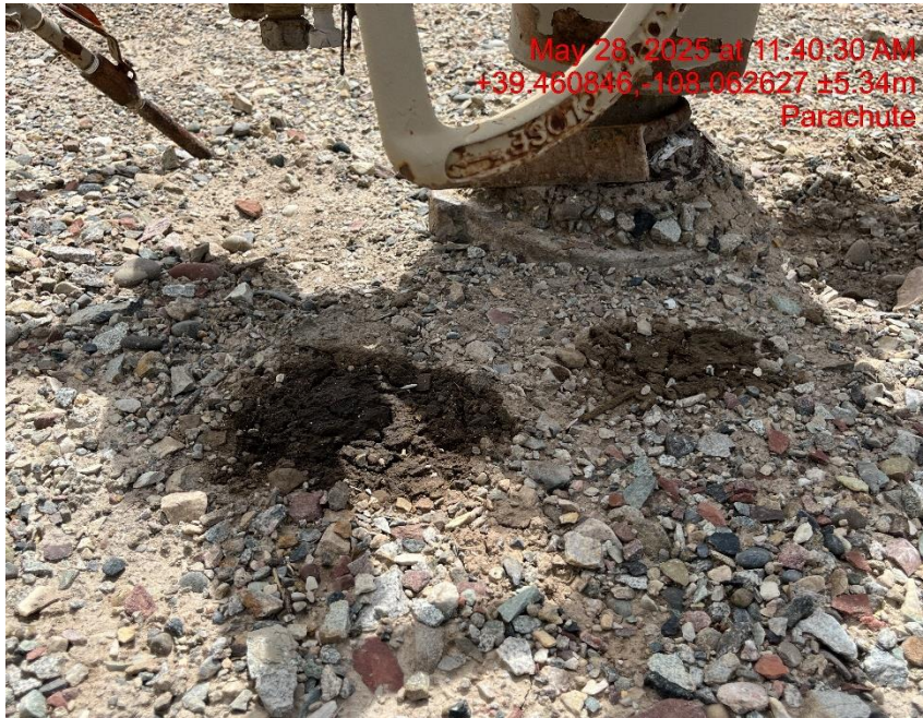
Photo # 7432 Small amount of staining at GM 324-1 wellhead
