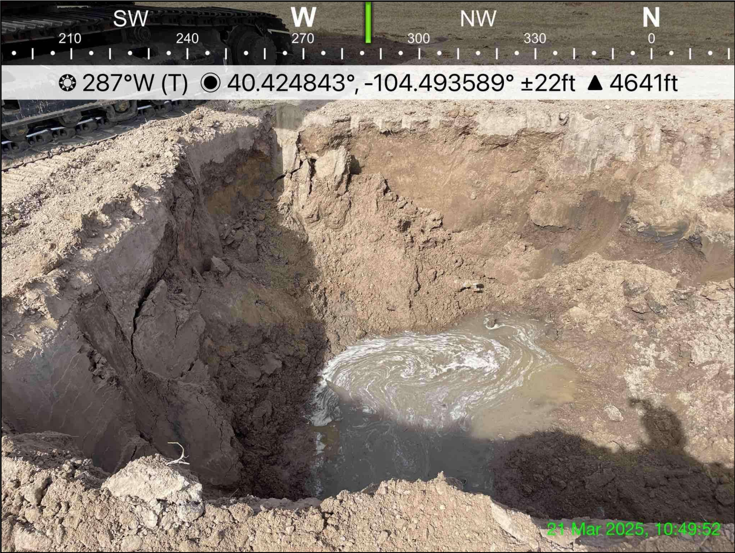
Photo 3: View of wellhead excavation with groundwater, facing west
