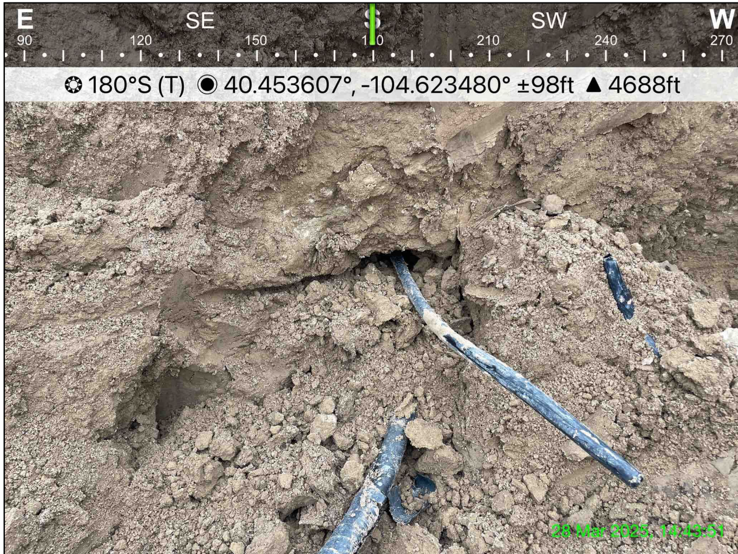
Photo 2: View of FL03-03 excavation area, facing south
