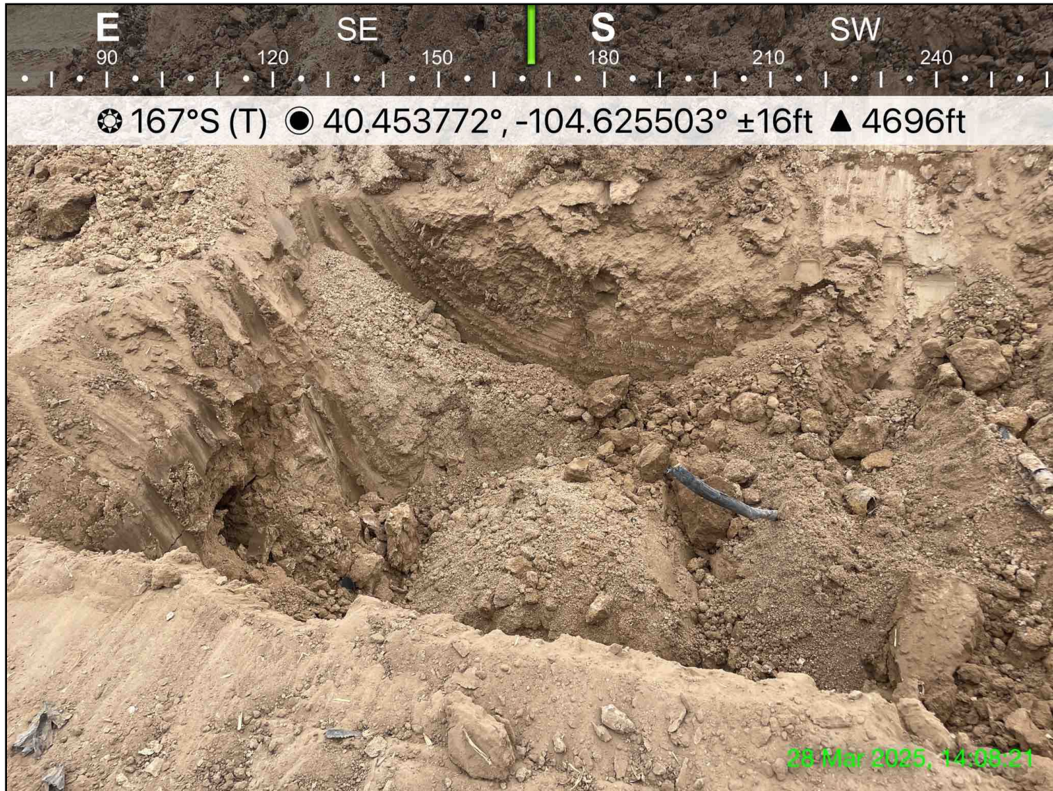
Photo 1: View of FL03-02 excavation area, facing south
