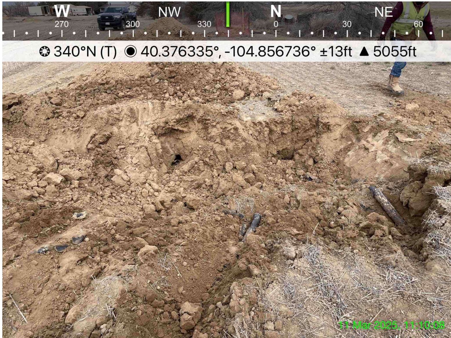
Photo 8: View of screening location PH03-FL01, facing northwest
