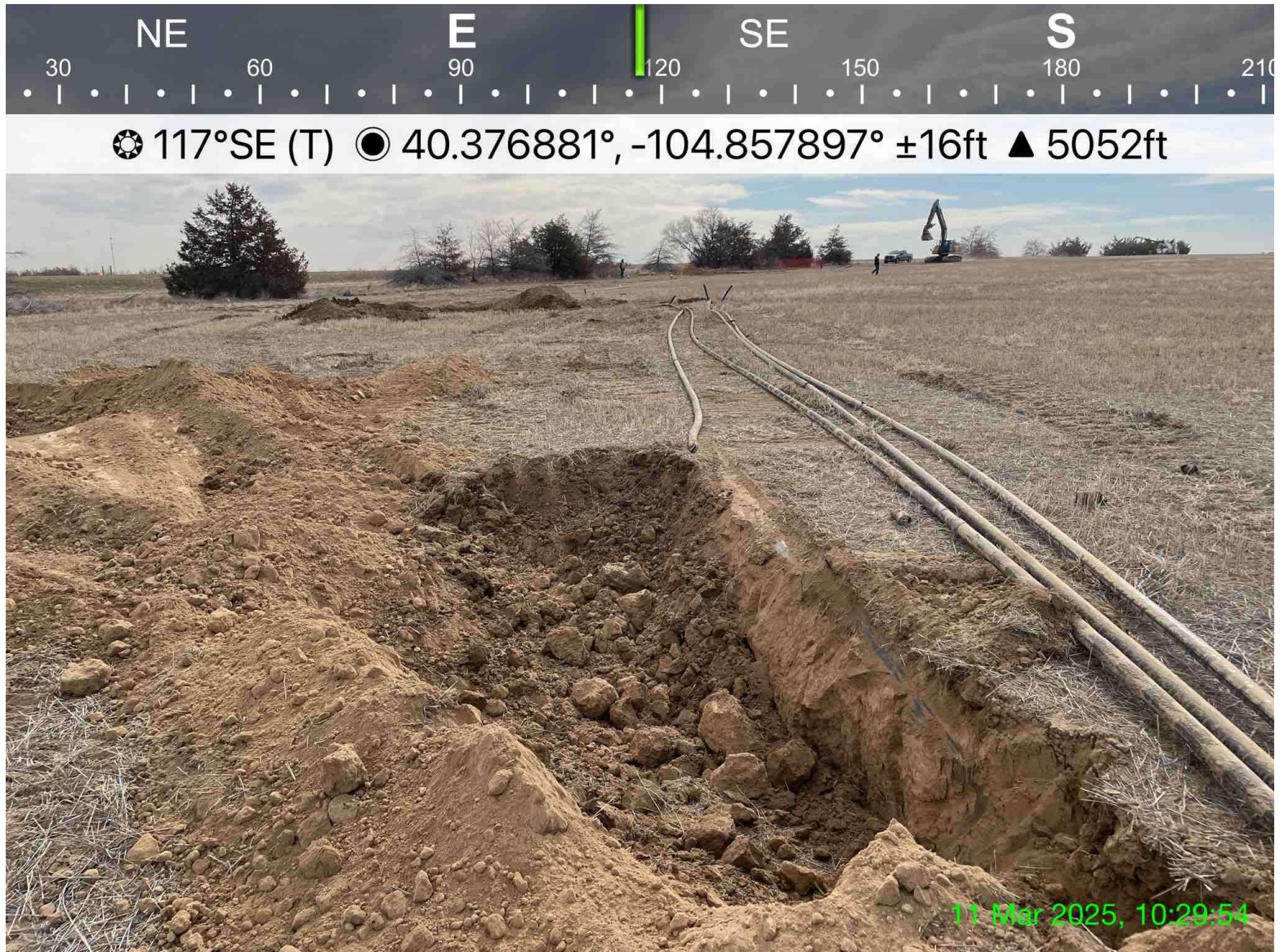
Photo 5: View of sampling location FL01-04, facing southeast
