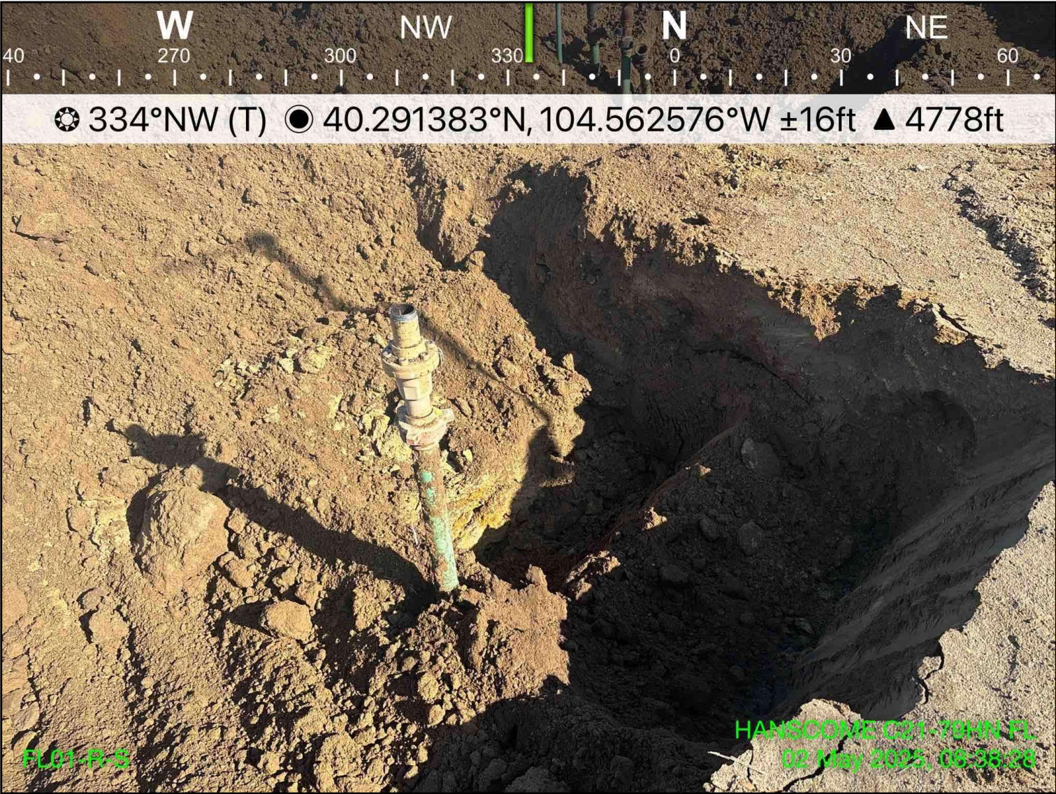
Photo 1: View of FL01-R-S, facing northwest
