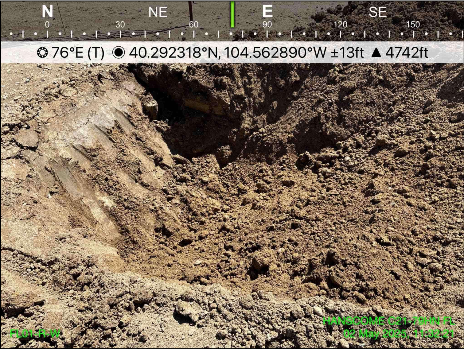
Photo 2: View of FL01-R-W, facing east
