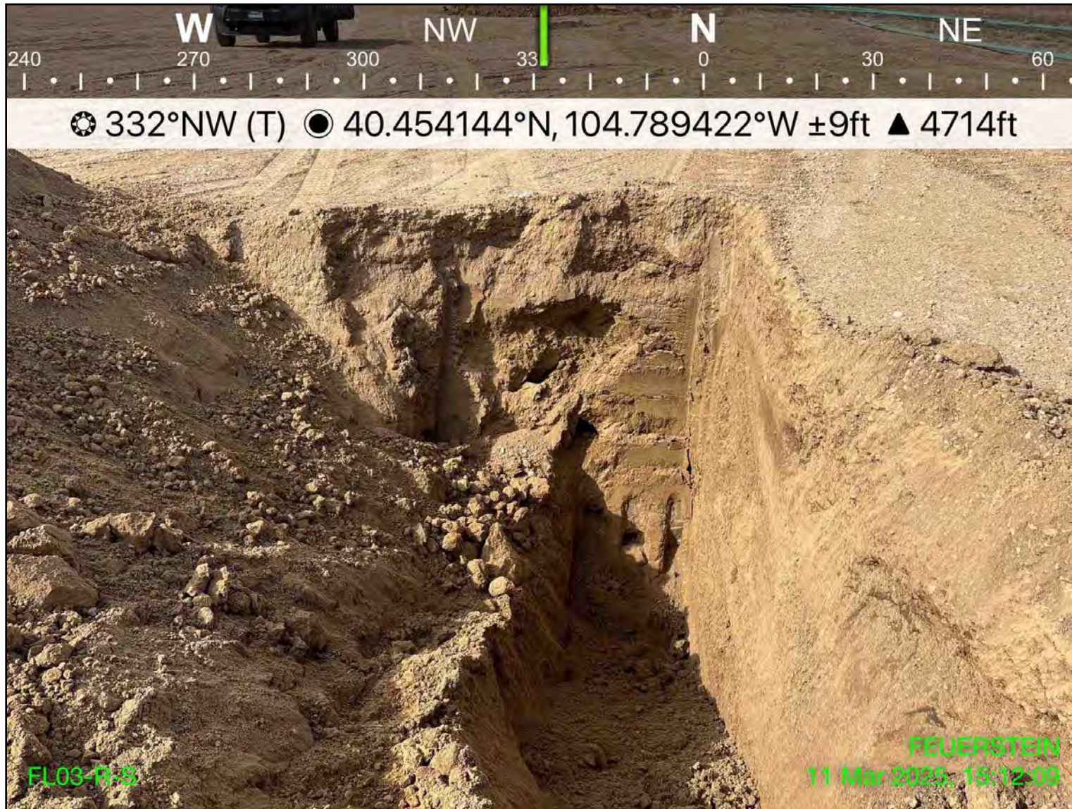
Photo 3: View of FL03-R-S, facing northwest
