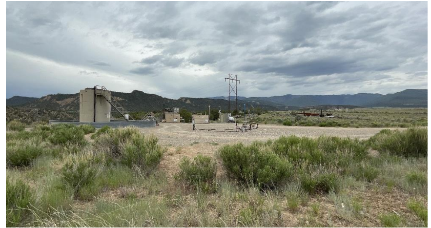
North East corner of location.
