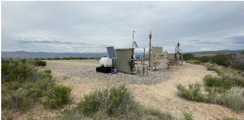
South West corner of location.
