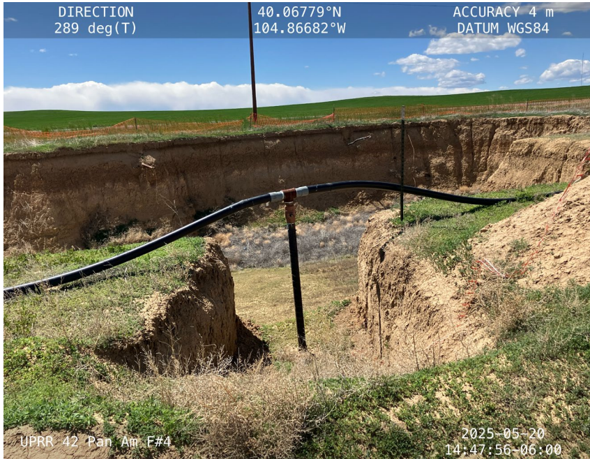
Flowlines appear to have been replaced with ~3" HDPE flowline pipe at the surface.
