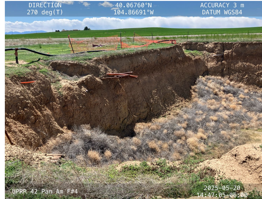
Excavation. Weeds. Torn fencing. Multiple flowlines of unknown status were observed exposed within the open excavation.
