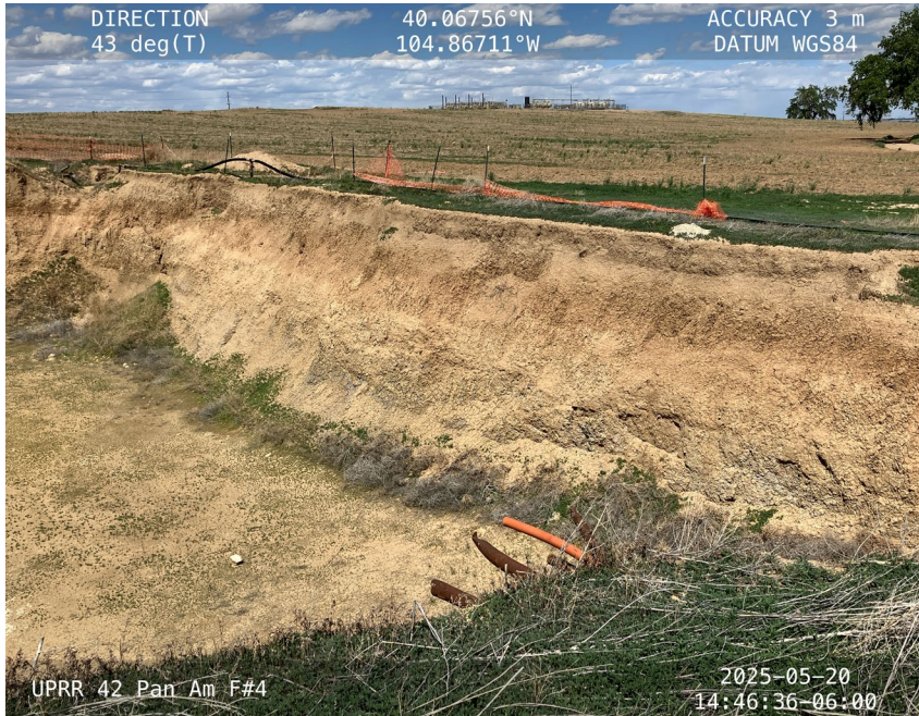
Excavation. Torn fencing. Multiple flowlines of unknown status were observed exposed within the open excavation.
