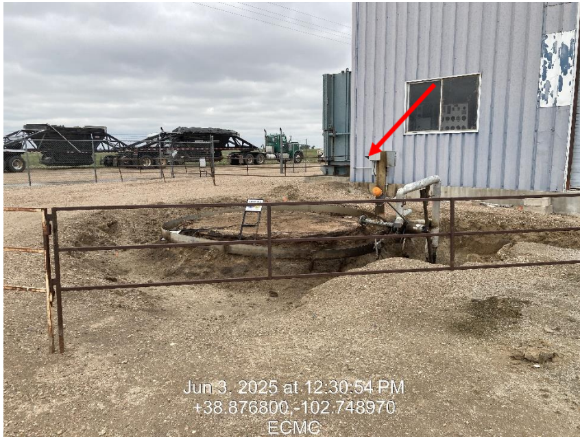
Photo 5 – Excavation area 2 at tank
