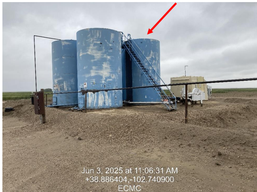
Photo 2 – Tank Battery
