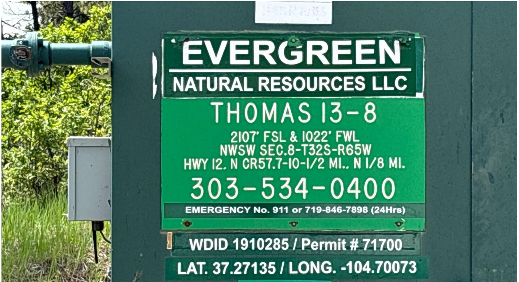
PHOTO 1: WELL SIGN HAS OLD EMERGENCY CONTACT NUMBER STILL VISIBLE AND API # IS NOT POSTED. Install sign to comply with Rule 605.a. CA DATE 7/4/2025.
