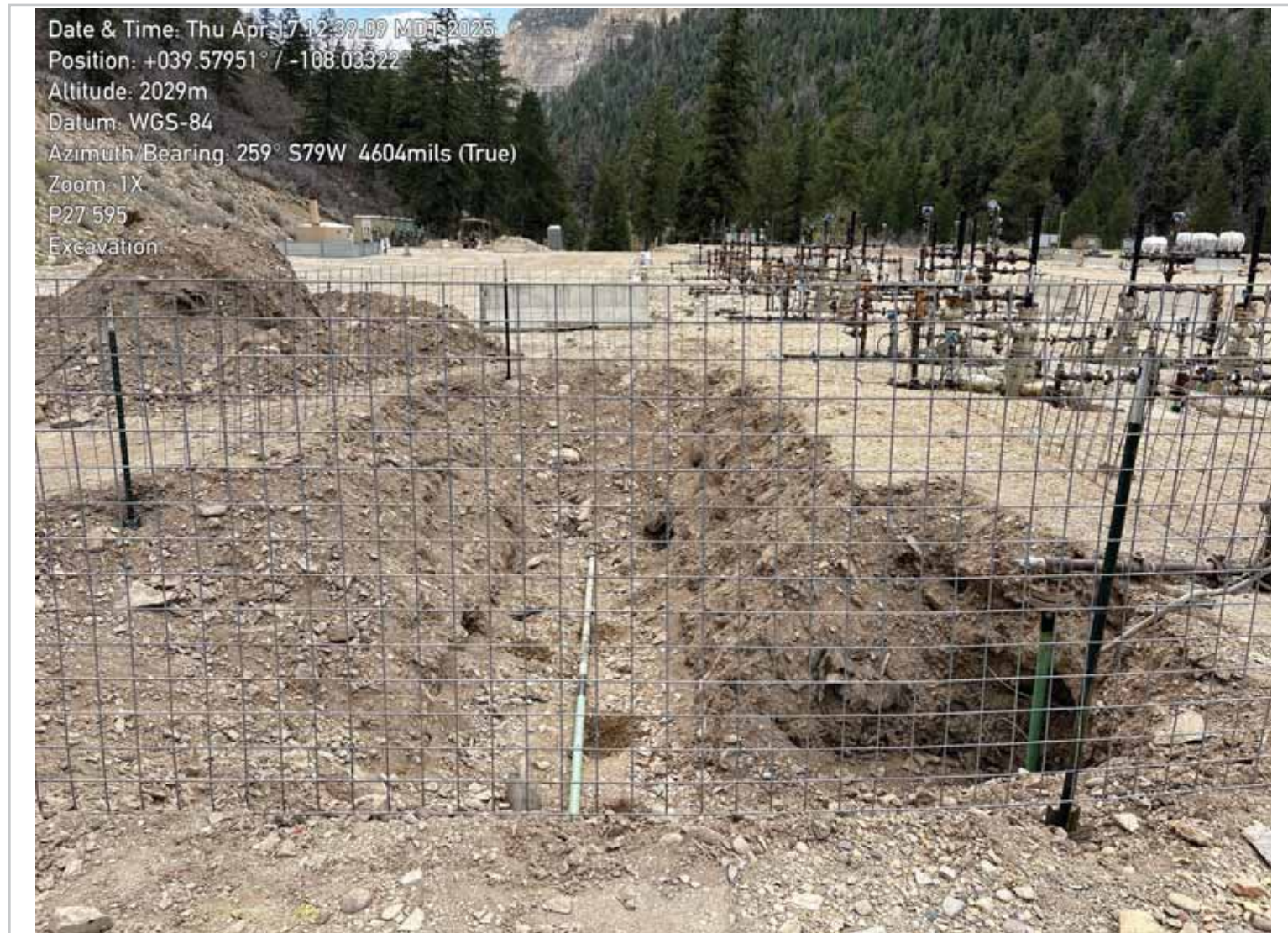
P27 595 16C-27 Excavation: View Southwest
