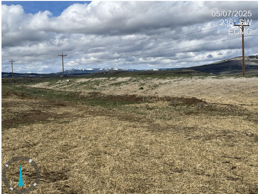
Photo 5. Photo taken from the northwestern portion of the location, facing topsoil stockpile. Topsoil has been stabilized with erosion matting.
