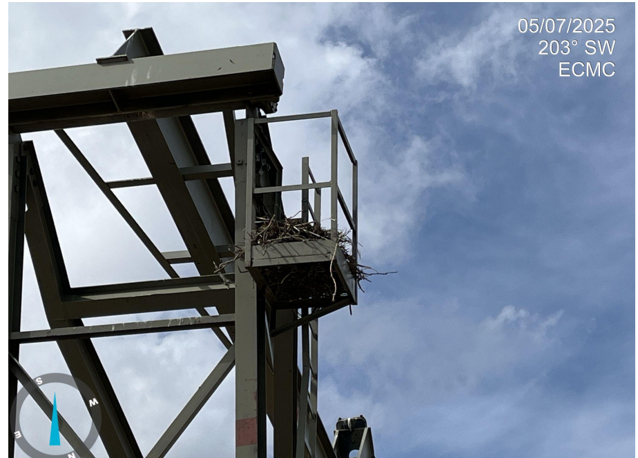
Photo 8. Photo taken at the northern side of the wellhead, illustrating an active bird nest on the pumpjack. Operator shall implement a work zone buffer and wait until fledglings are no longer present to continue operations pursuant to Rule 902.b.
