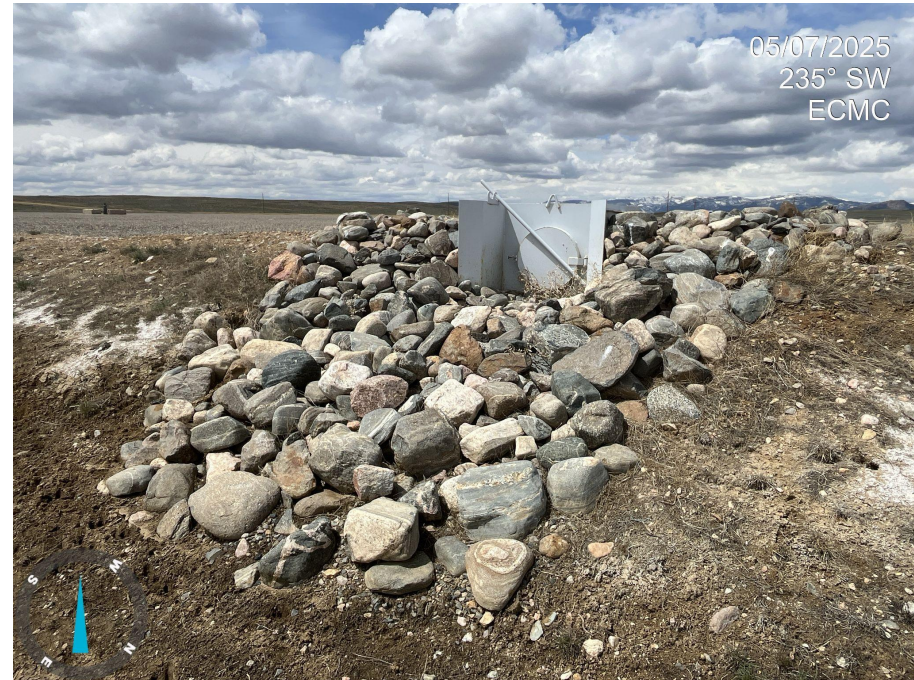
Photo 8. Photo taken at the eastern portion of the Location, facing the stormwater outlet. It is unclear if geotextile lining has been installed under the riprap per good engineering practices.
