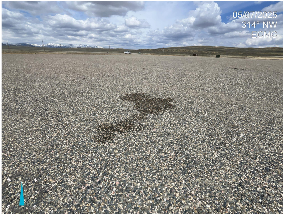
Photo 11. Photos 11-12 illustrate stained/impacted soils observed throughout areas on the pad. Remove and properly dispose of impacted material.
