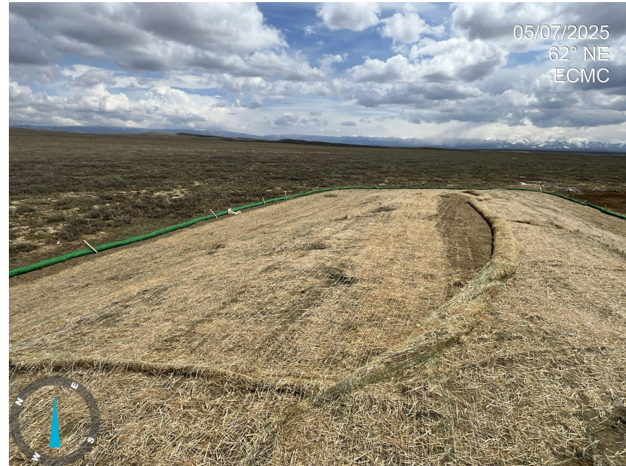
Photo 6. Photo taken of the topsoil stockpile. Maintain erosion matting to prevent degradation of the topsoil stockpiles.
