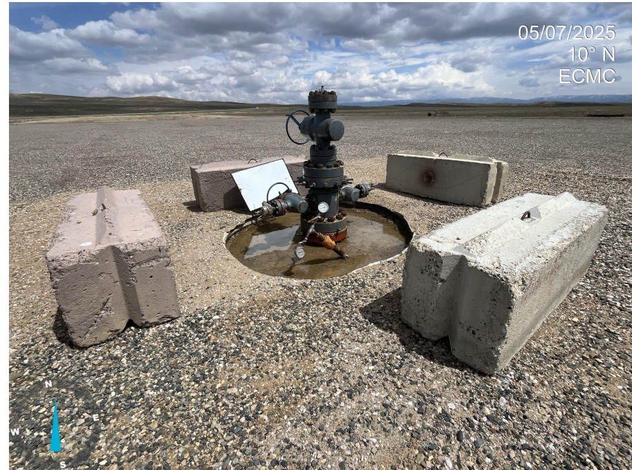
Photo 4. Photo taken at the wellhead. The photo illustrates ponding water in the wellhead cellar.
