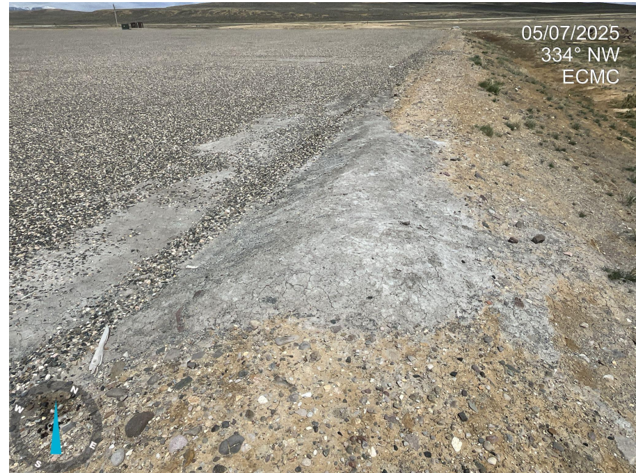
Photo 10. Photo taken at the southeastern portion of the Location. What appears to be cement waste has spilled on the location and perimeter berm.
