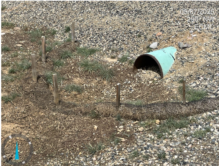
Photo 3. Photo illustrates culvert at the entrance of the Location. No erosion issues observed at this time. However, the culvert does not appear to have been installed with inlet/outlet protections per good engineering practices.
