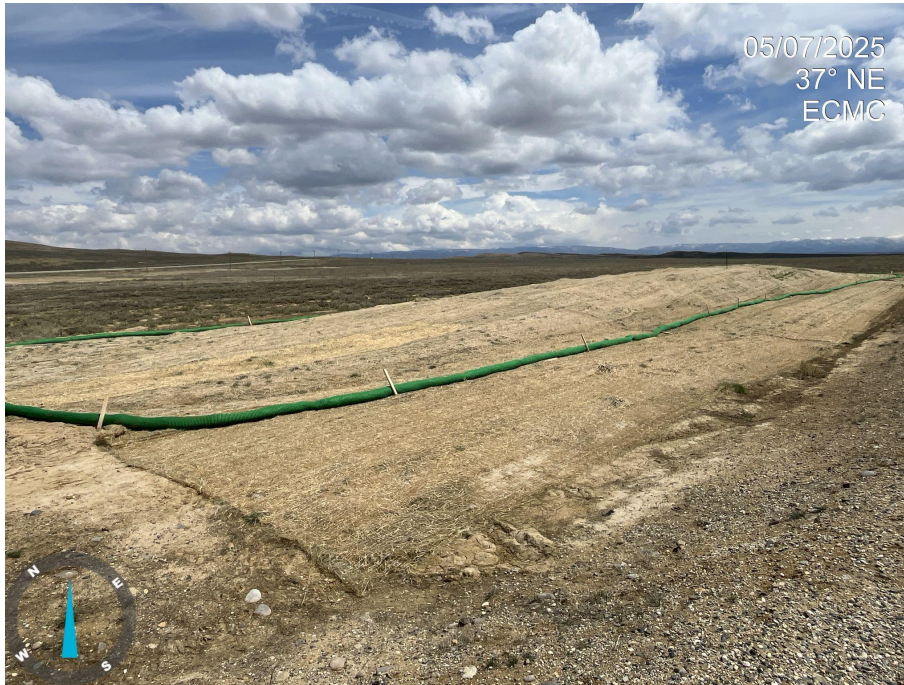
Photo 5. Photo taken of the topsoil stockpile. At this time, it does not appear enough topsoil was salvaged at the time of construction per 1002.b.
