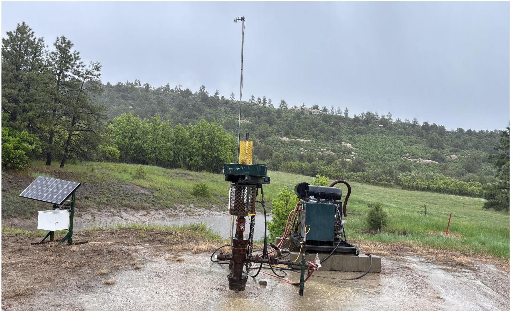
PHOTO 3: WELLHEAD AND EQUIPMENT.
