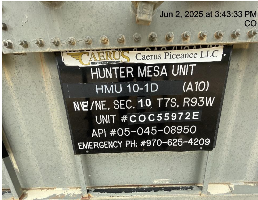
Photo # 5444 Emergency contact # on wellhead sign incorrect/# is disconnected & not in service
