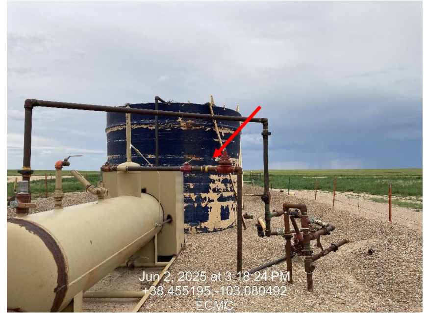
Photo 6 – Leaking valve repaired
