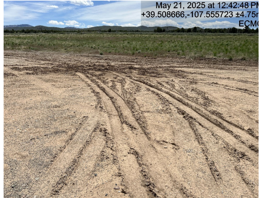
Lack of stabilization with out any tracking controls
