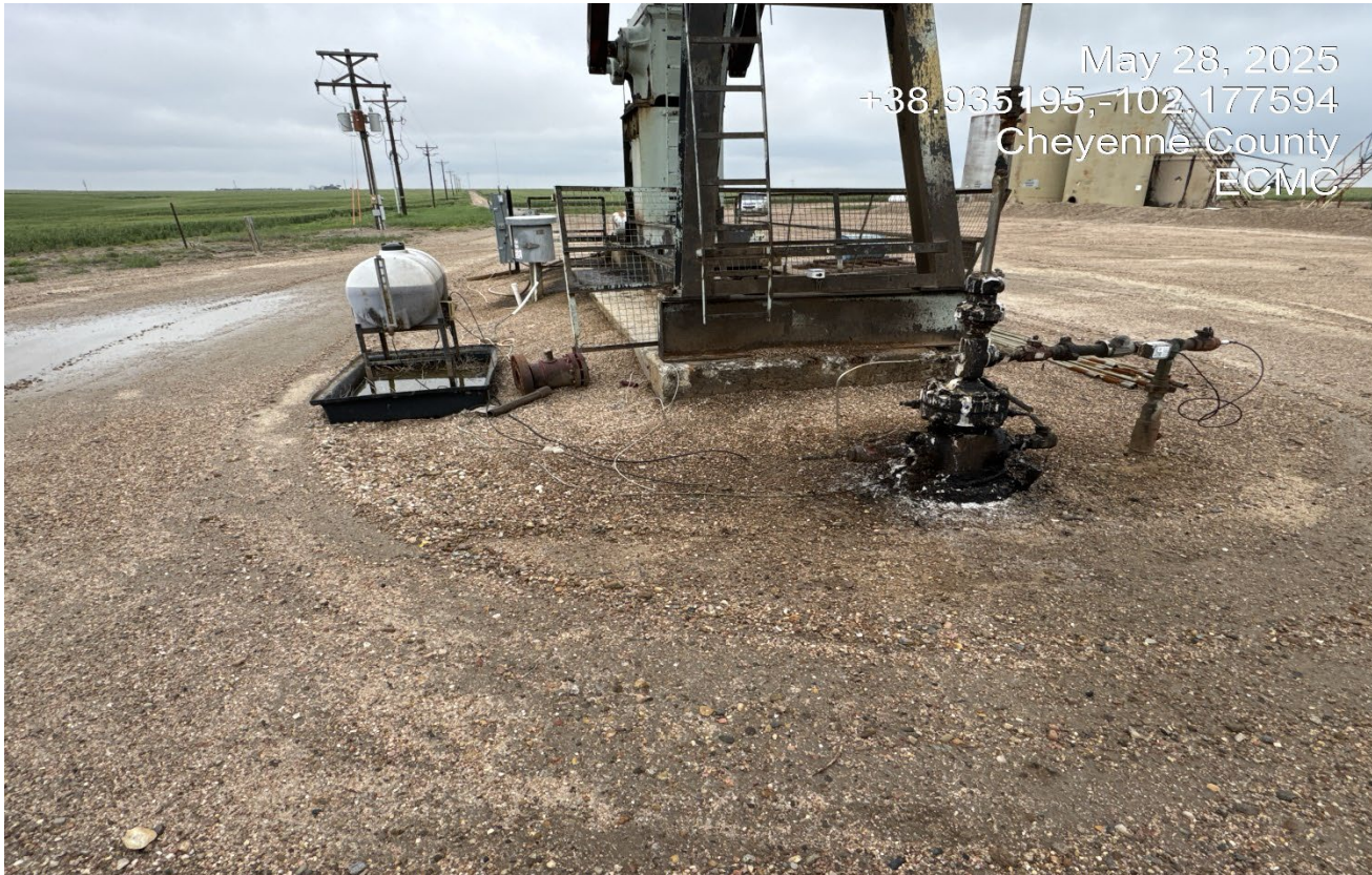
Photo 5. There is stained soils at the wellhead that need to be cleaned up and properly disposed. There is a leak at the wellhead that needs to be fixed.
