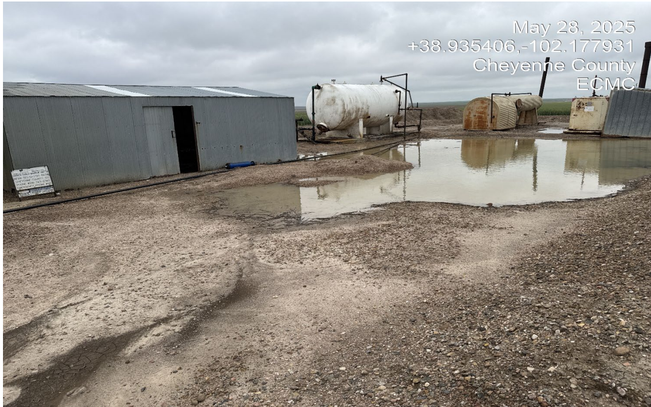
Photo 8. Facing northeast at the tank battery facility. Sign has been installed.
