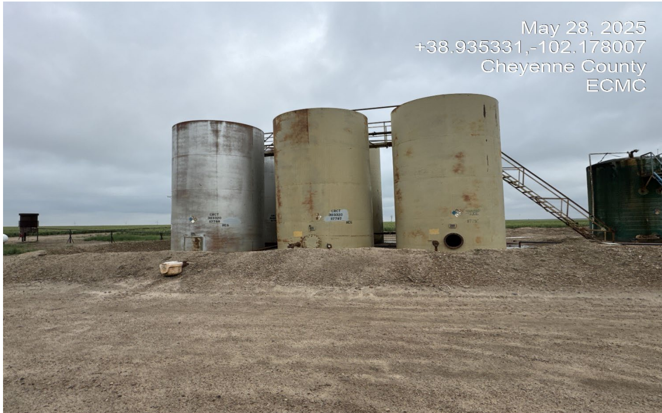
Photo 7. Facing toward the tank battery. Some of the labels are faded and missing information.
