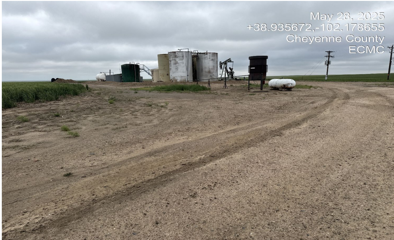
Photo 1. Facing southeast toward the tank battery.
