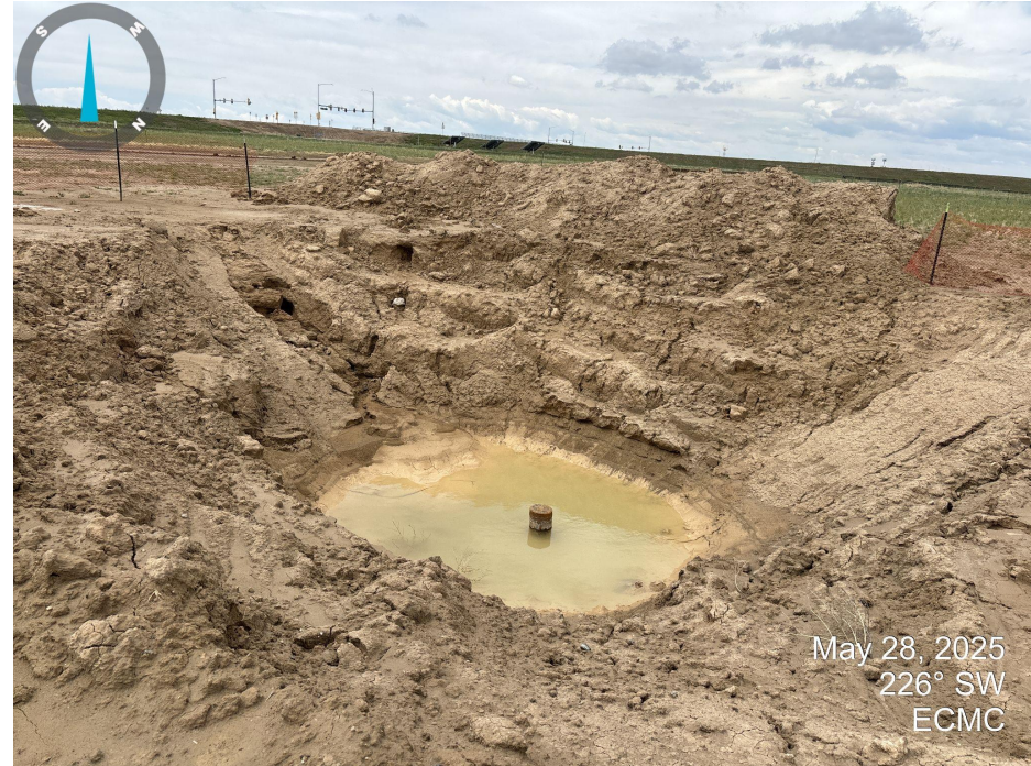
Photo 4. The wellhead is visible at the bottom of the excavation. Erosion is present inside of the excavation and on the soil piles.
