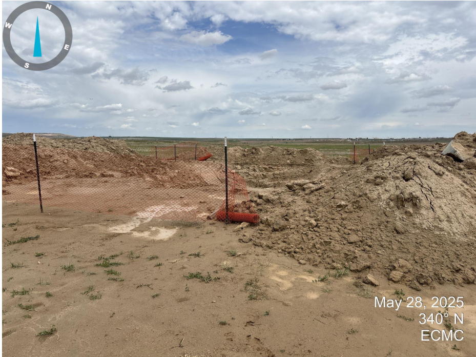
Photo 3. Construction fencing does not appear to be adequately installed to prevent entry. Soil piles do not appear to have any liners or stabilization.
