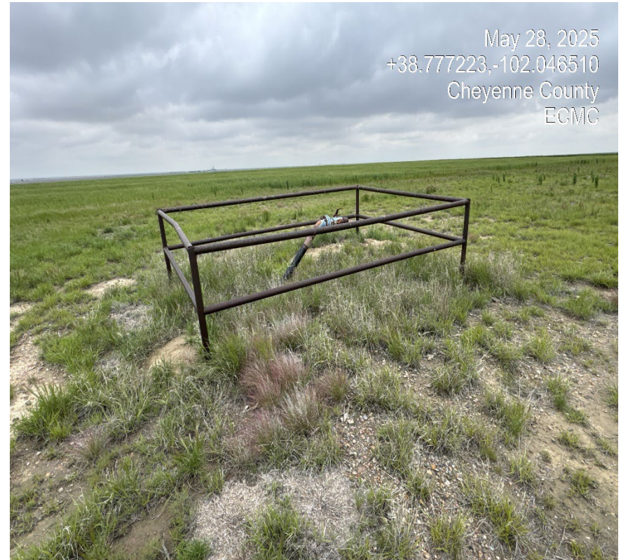
Photo 5. Photo of pipe riser that remains at the former tank battery.
