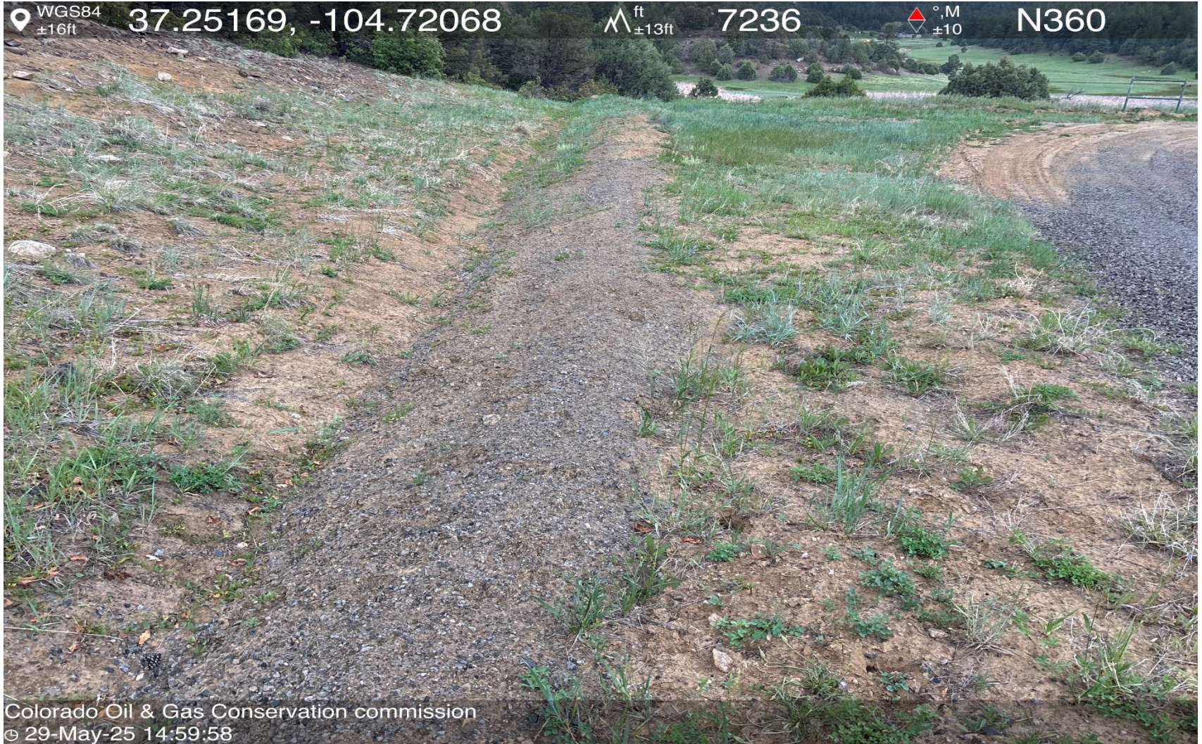
PHOTO 5: THE DOWNSLOPE SIDE OF CULVERT IS COMPLETELY COVERED.
