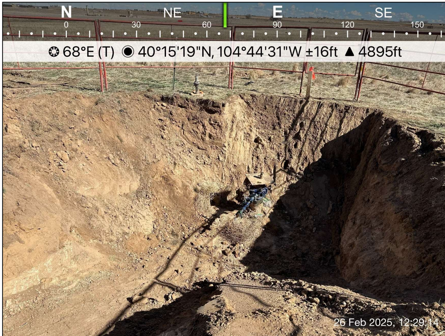
Photo 4: View of excavation, facing northeast-east
