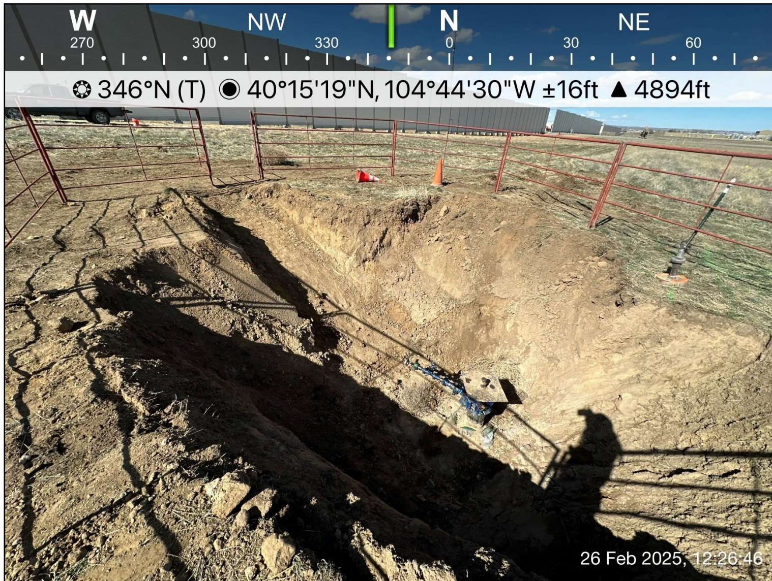
Photo 3: View of excavation, facing north-northwest
