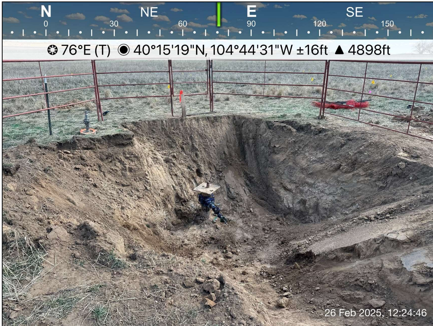
Photo 1: View of excavation, facing northeast-east
