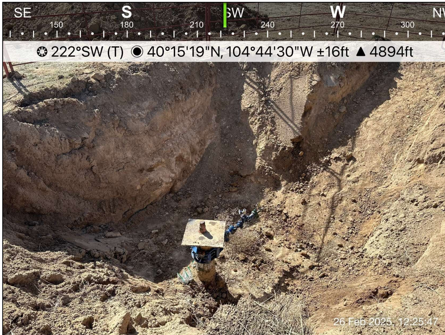
Photo 2: View of excavation, facing southwest
