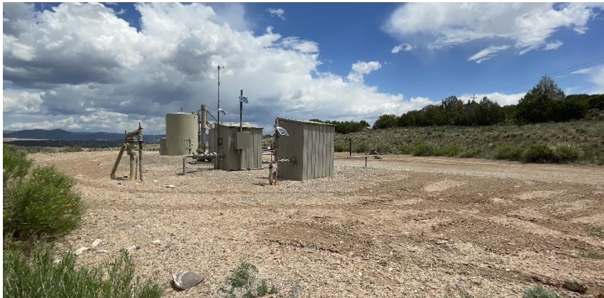
South West corner of location.
