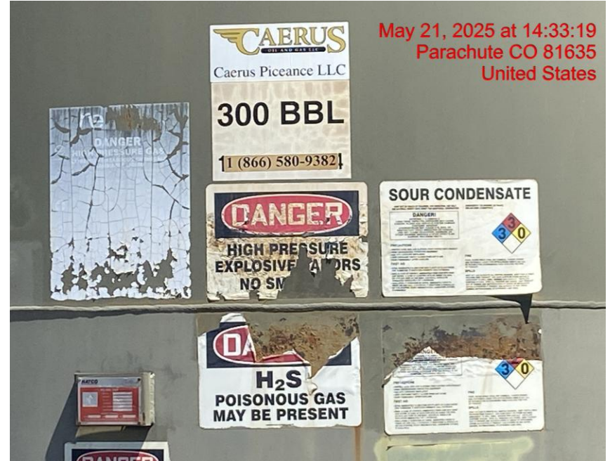
Weathered/Unserviceable Tank Labels – Photo #08980
