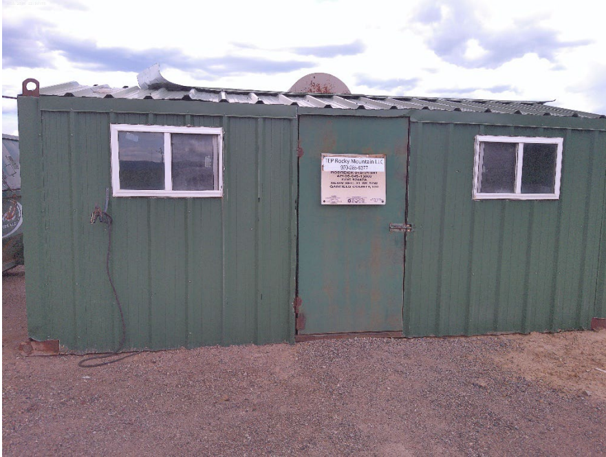
Injection wellhead inside housing
