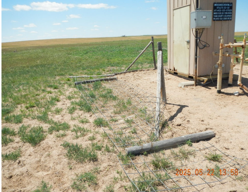
5. View of fencing at metering location.
