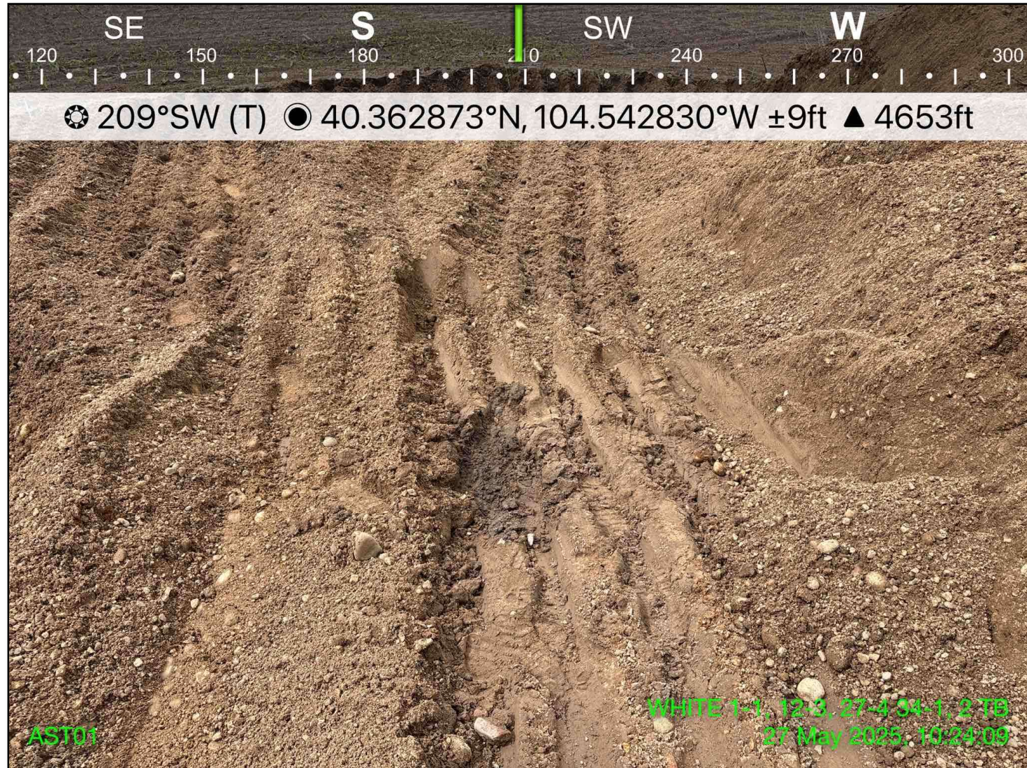
Photo 1: View of AST01 excavation area, facing southwest
