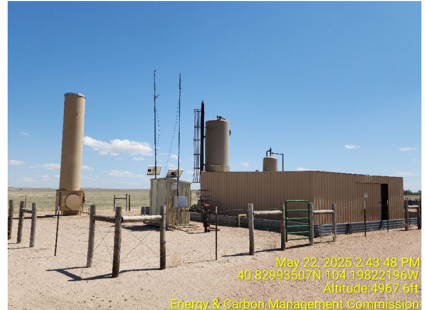
Photo 2 – Heater Treater, ECD and Gas Meter
