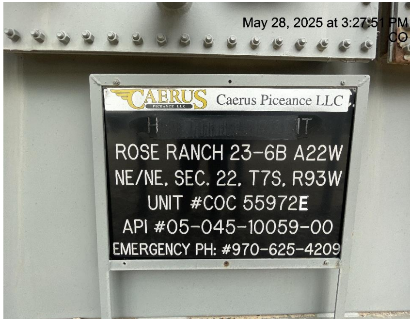
Photo # 3782 Emergency contact # on wellhead sign incorrect/# is disconnected & not in service
