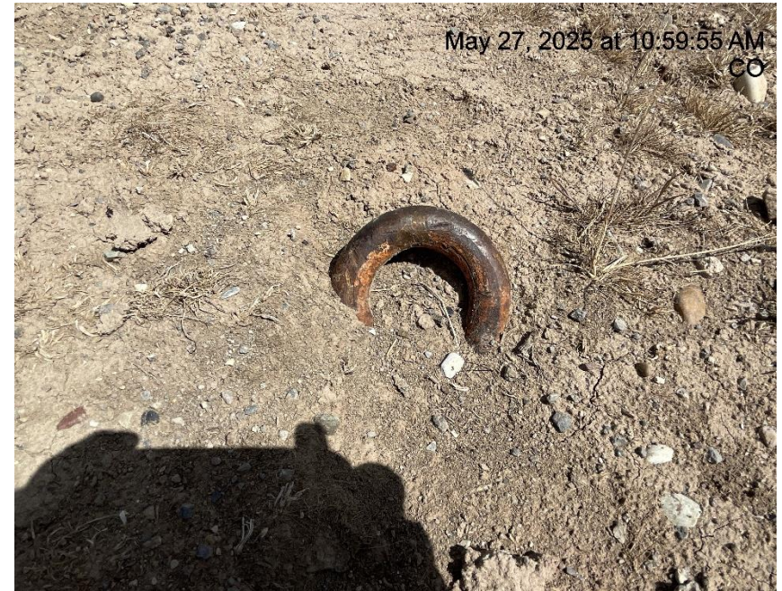
Photo # 3445 Unmarked deadman
