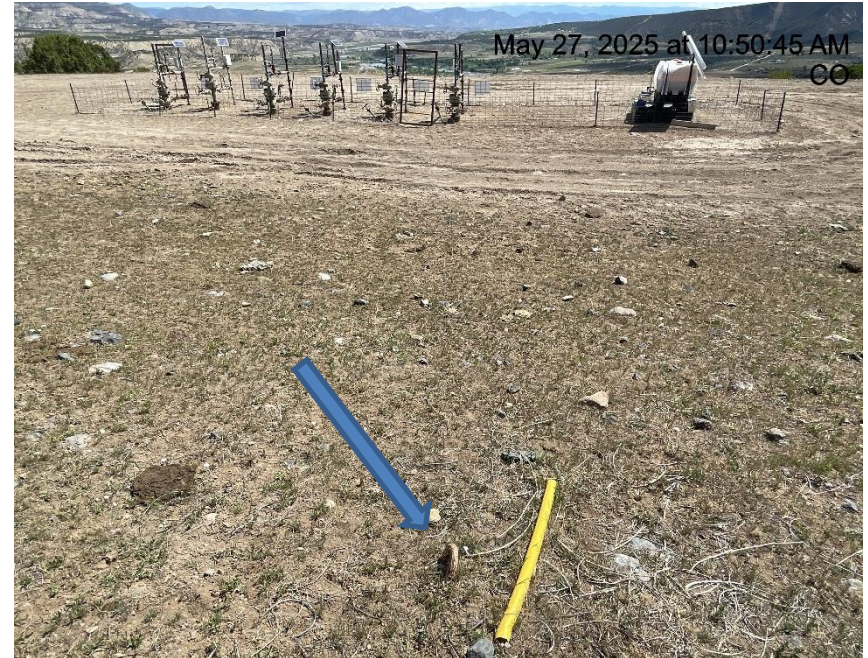
Photo # 3449 Same improperly marked deadman
