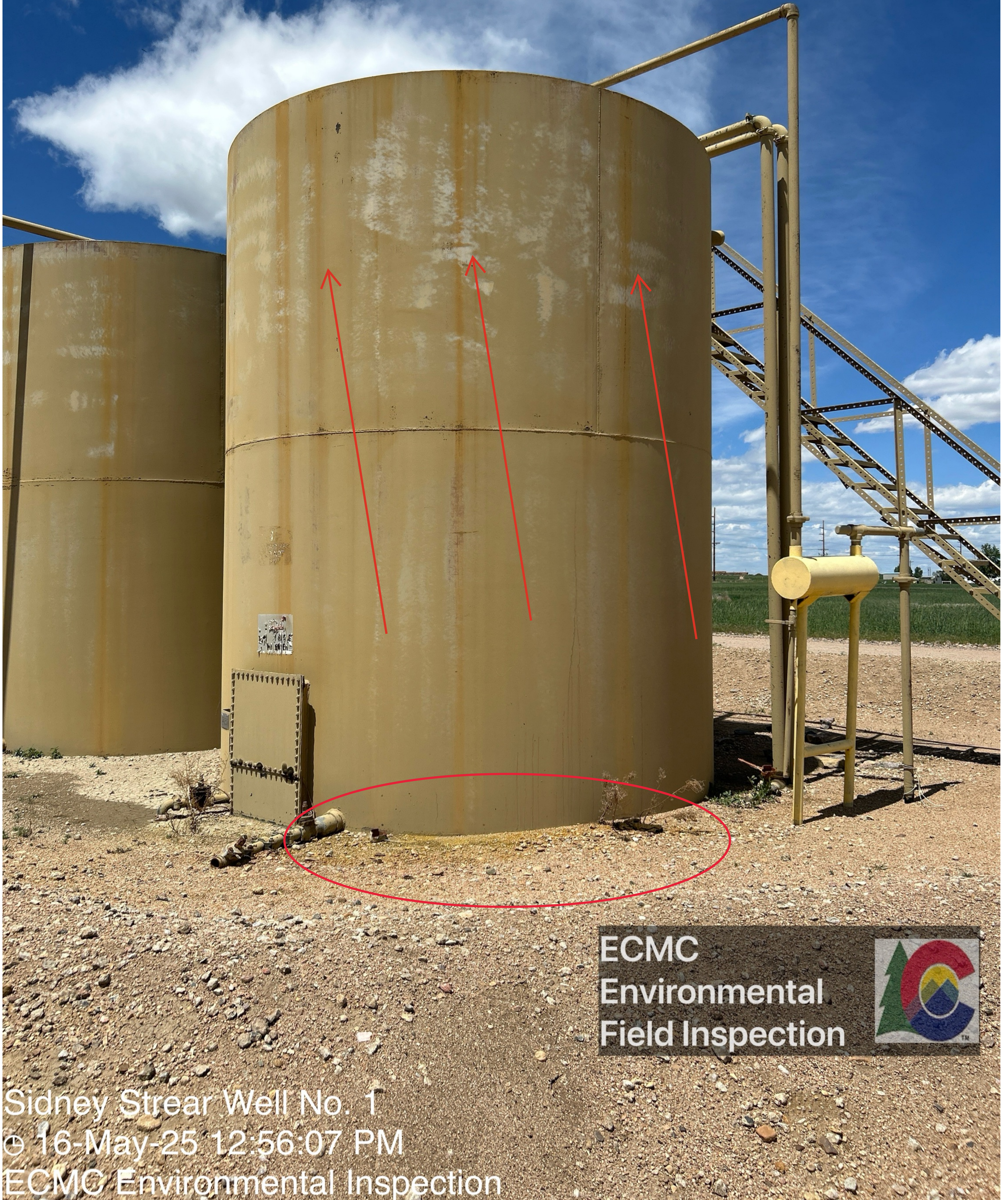
Yellow-stained soil is visible at the base of the production tank. Rust is visible on the side of the production tank.
