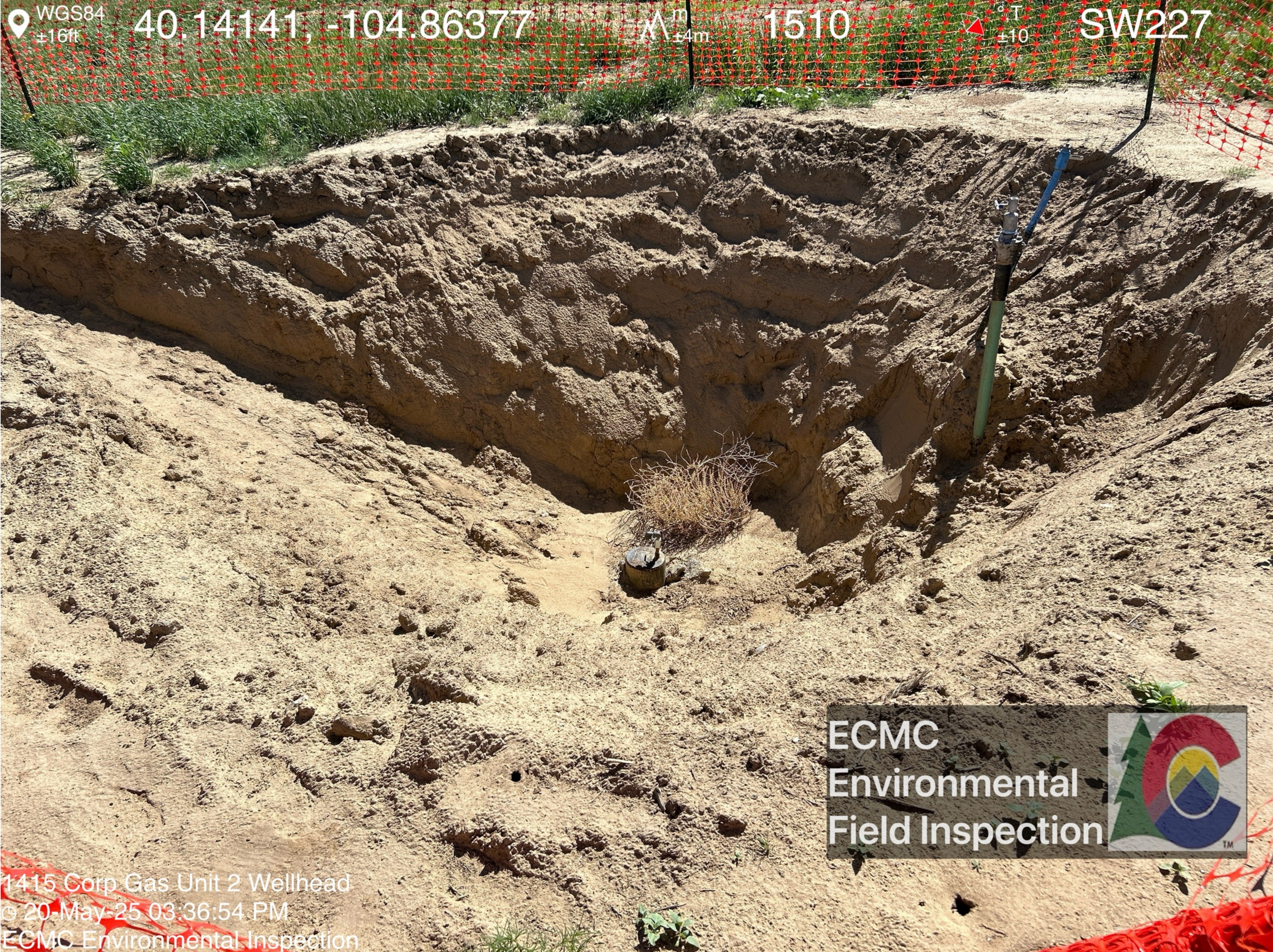
Two risers are visible within the excavation. Debris is visible at the base of the excavation.
