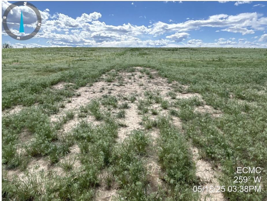
Photo 5. Photo taken from the access road, facing West towards the well location. Photo illustrates that final reclamation activities appear to have taken place, but vegetation has not established to Rule 1004 standards. Cheatgrass ( Bromus tectorum ) is present across the access road and is a List C noxious weed species.
