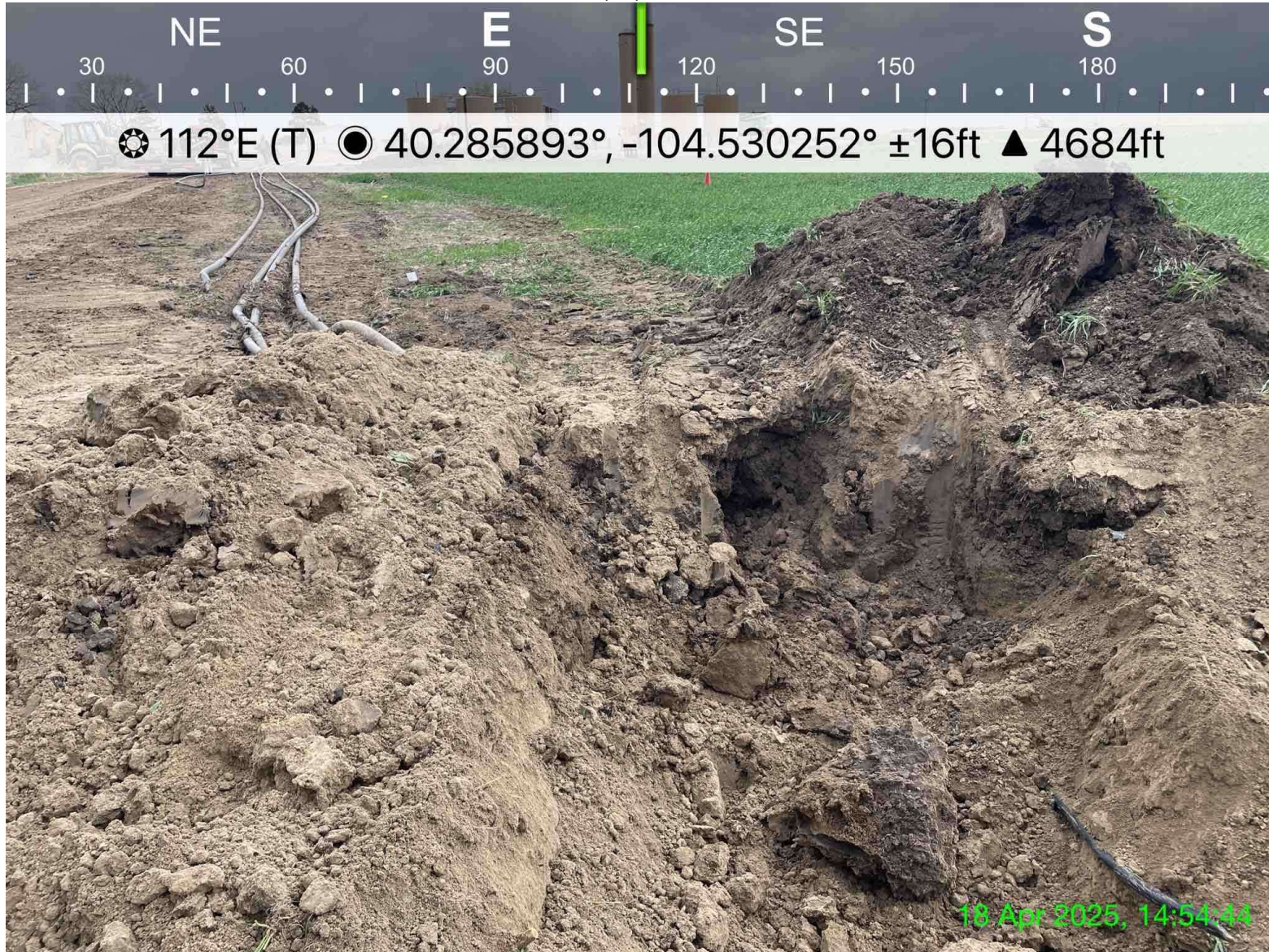
Photo 7: View of PH19 screening location, facing east
