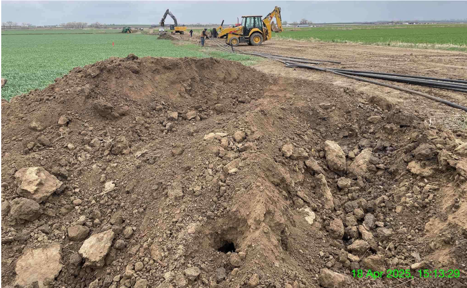
Photo 8: View of FL02-06 sampling location, facing west
