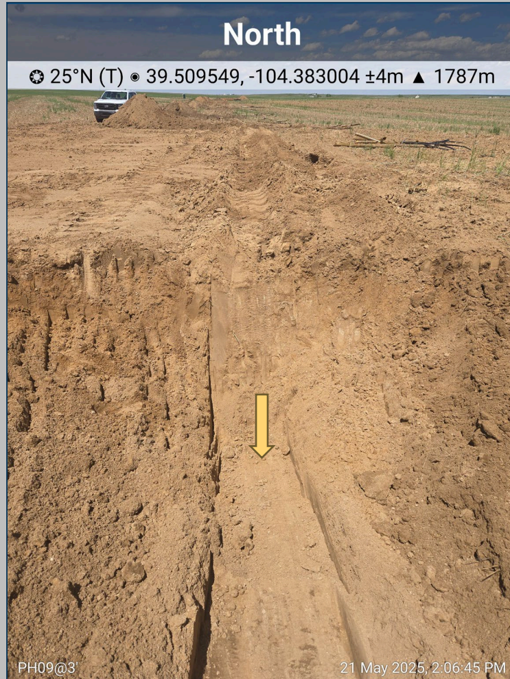
Flowline Pothole Soil Screen PH09@3'
