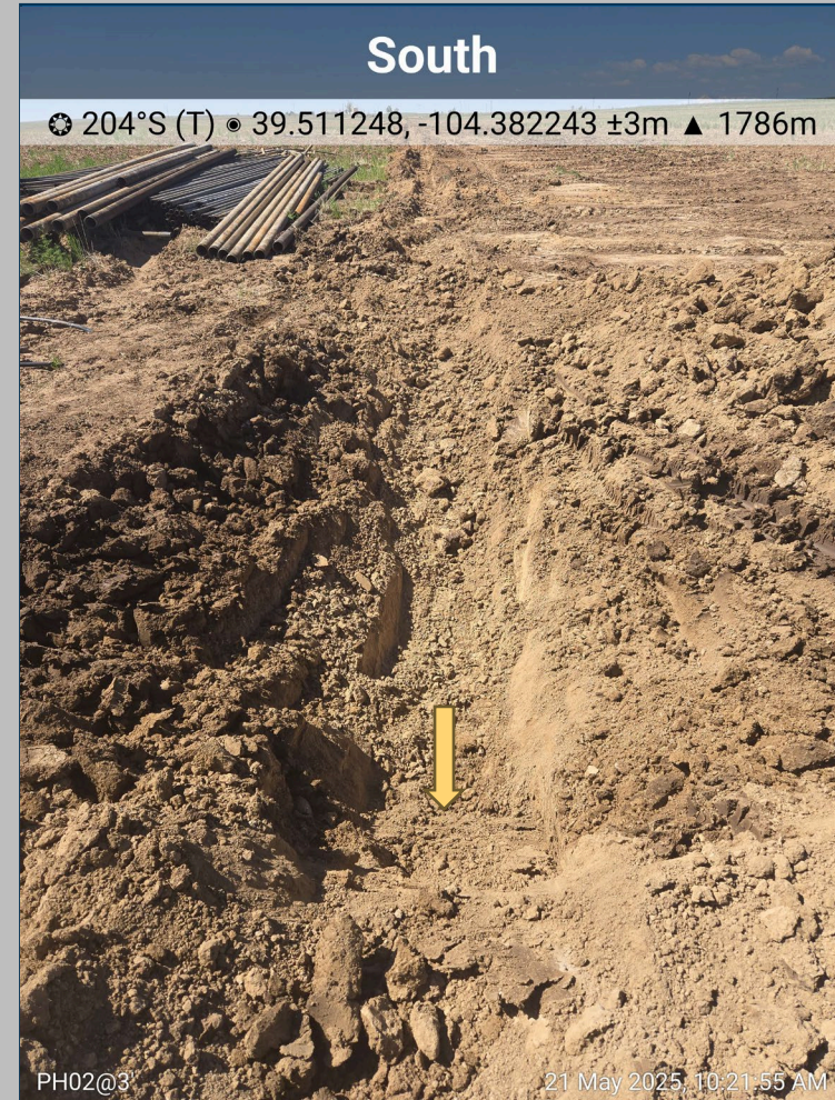
Flowline Pothole Soil Screen PH02@3'
