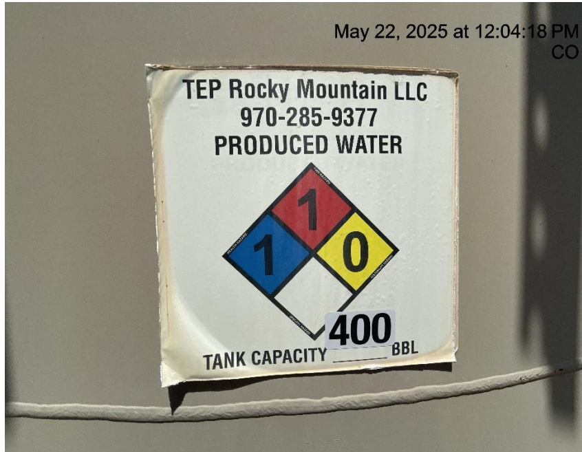
Photo # 2308 Tank capacity incorrect
