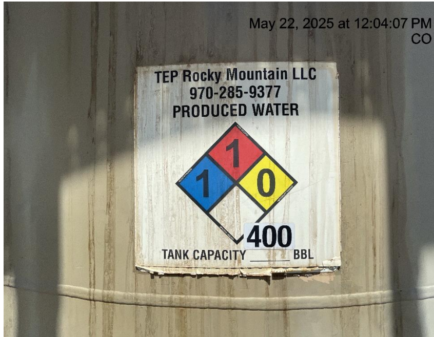
Photo # 2306 Tank capacity incorrect
