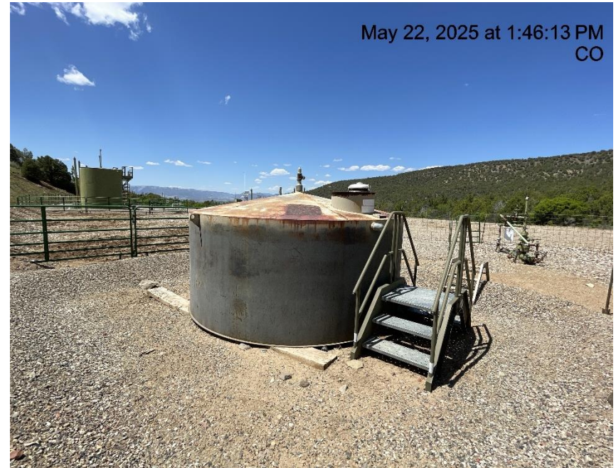
Photo # 2835 Tank is disconnected & not in use/unused equipment
