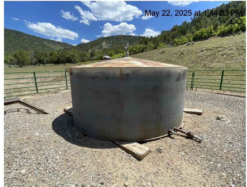
Photo # 2834 Tank is disconnected & not in use/unused equipment
