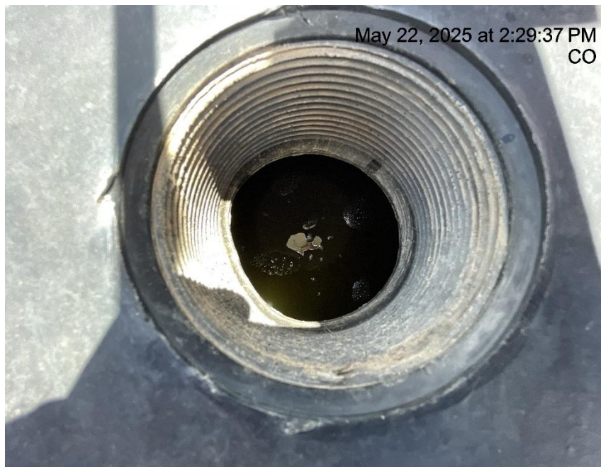
Photo # 3001 Failure to maintain chemical BMP - Chemical tank containment approximately 2/3 to 3/4 full of fluid/BMP insufficient to contain possible spill
