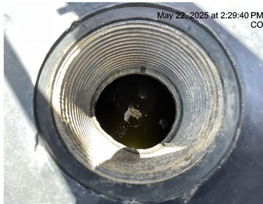
Photo # 3002 Failure to maintain chemical BMP - Chemical tank containment approximately 2/3 to 3/4 full of fluid/BMP insufficient to contain possible spill
