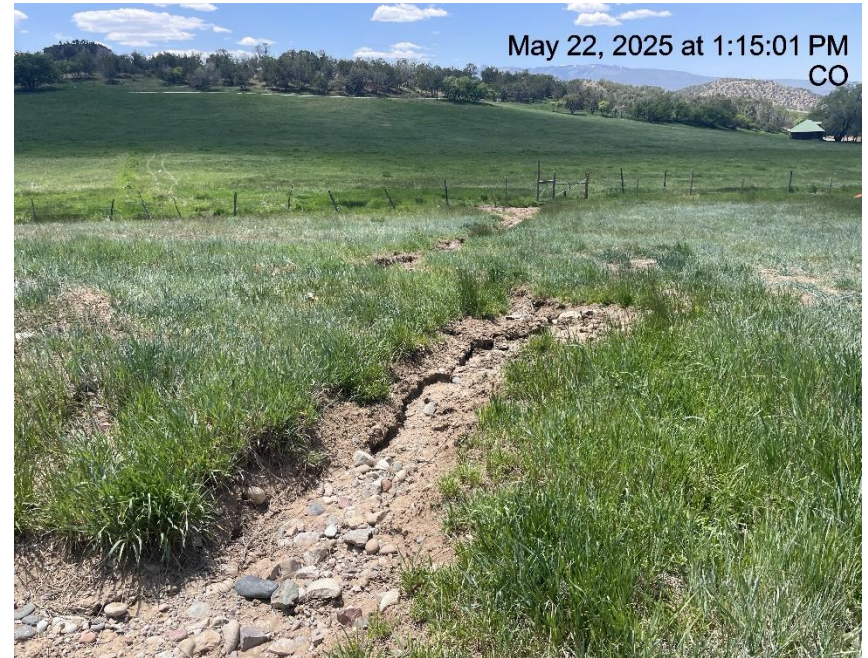
Photo # 2482 Failure to minimize erosion & transport of sediment off location/insufficient BMP's
