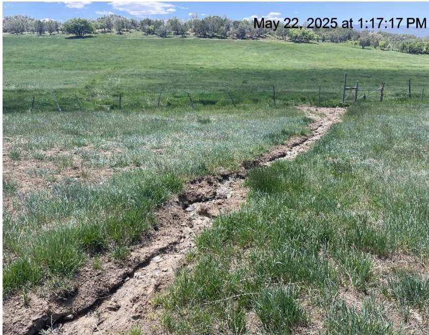
Photo # 2483 Failure to minimize erosion & transport of sediment off location/insufficient BMP's
