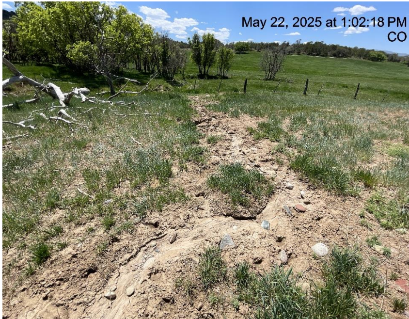
Photo # 2473 Failure to minimize erosion & transport of sediment off location/insufficient BMP's
