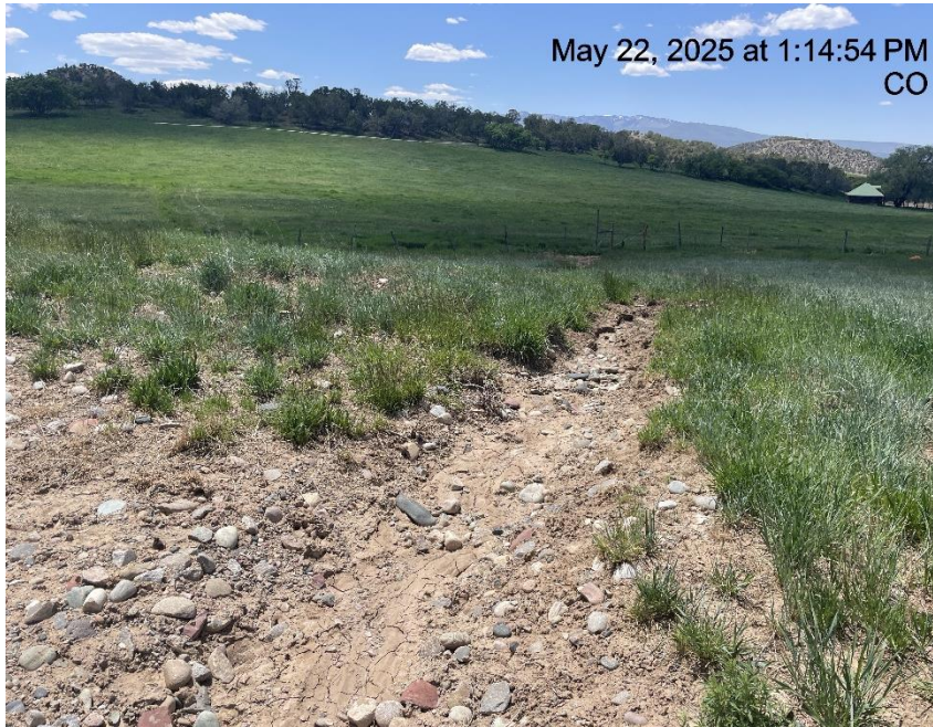
Photo # 2481 Failure to minimize erosion & transport of sediment off location/insufficient BMP's
