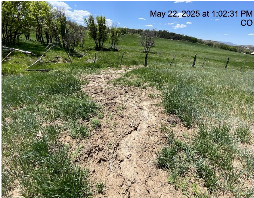
Photo # 2475 Failure to minimize erosion & transport of sediment off location/insufficient BMP's
