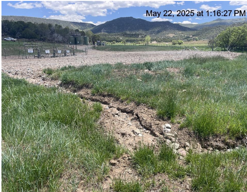
Photo # 2479 Failure to minimize erosion & transport of sediment off location/insufficient BMP's
