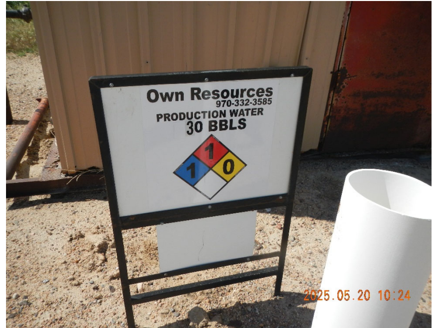
4. Content/Quantity/Hazard sign at produced water tank.
