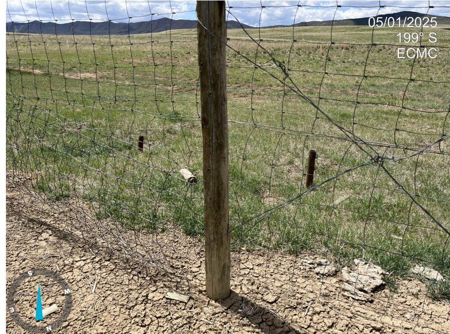
Photo 10. Photo taken from the west end of the pit facility, facing south. Photo illustrates anchor pipes, which have not been properly covered to prevent wildlife access, including birds and bats.
