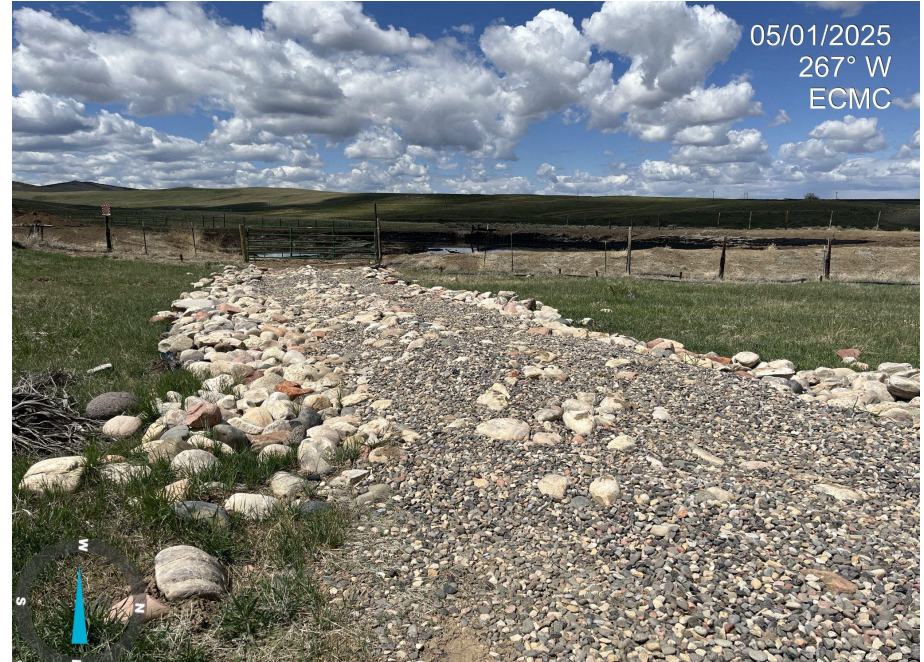
Photo 4. Photo taken from the east end of the pit facility outside of the fence, facing west. Photo illustrates track-out controls not installed per good engineering practices; BMP has been installed with small gravel material, rather than larger sized coarse aggregate. Repair/install tracking BMPs.
