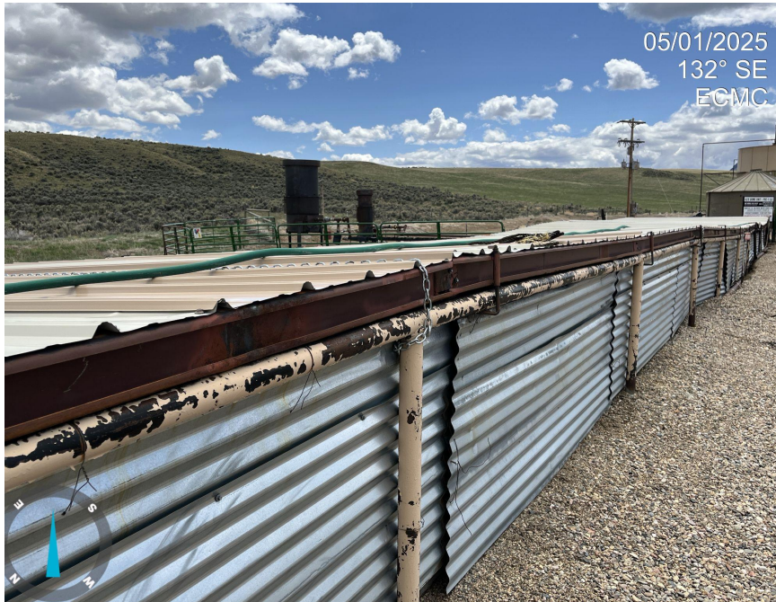
Photo 32. Photo taken from northern portion of Tank Battery facility, facing southeast. Photo shows overview of the covered pit.
