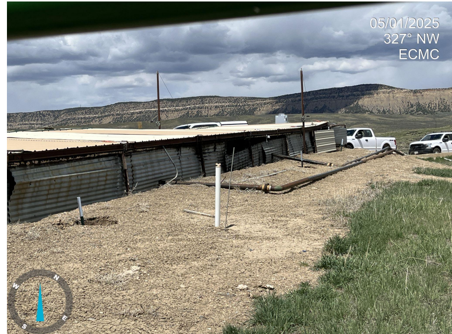
Photo 33. Photo taken from northeast portion of Tank Battery facility, facing northwest. Photo shows overview of covered pit.
