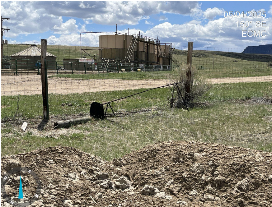
Photo 7. Photo taken from the south end of the pit facility, facing southeast. Photo illustrates trash/debris.
