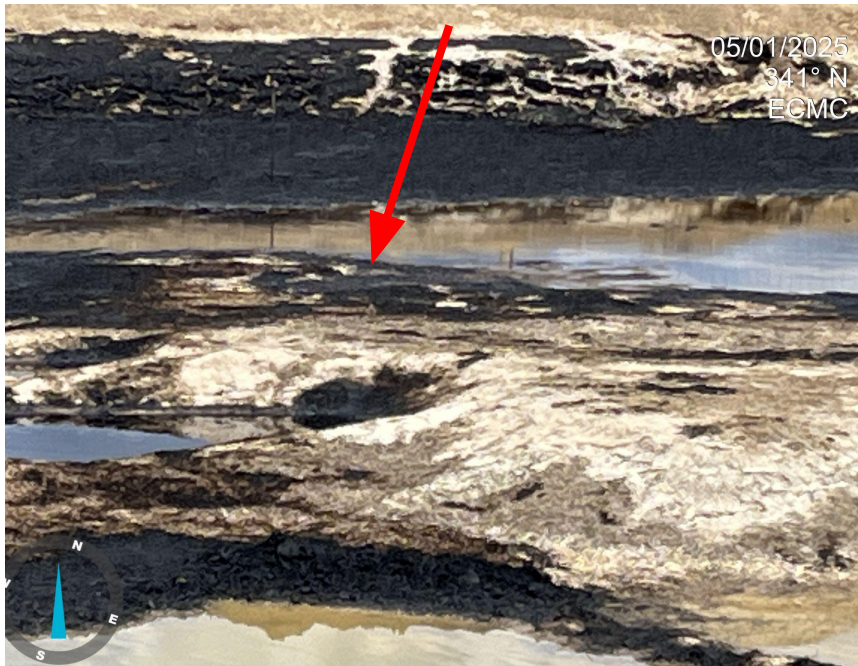
Photo 30. Photo taken from the south end of the pit facility, facing north. Photo illustrates lack of wildlife protection, allowing wildlife access to the pit (red arrow indicates killdeer landing on pit).
