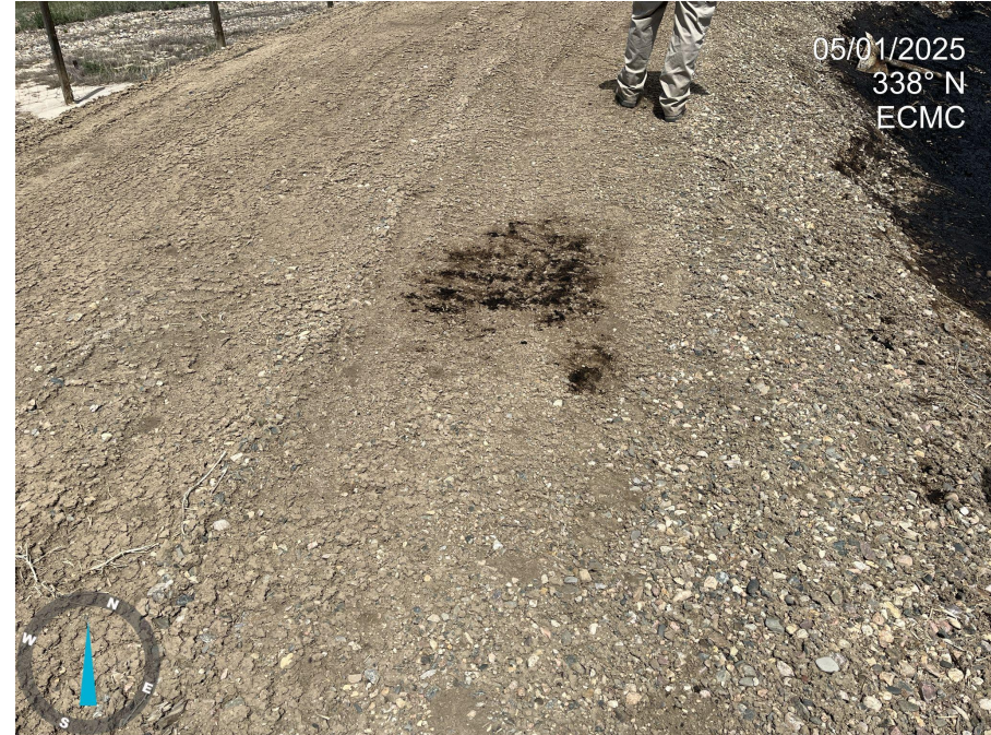
Photo 16. Photo taken from the west end of the pit facility, facing north. Photo example showing stained/impacted soils observed throughout areas of the pit facility.
