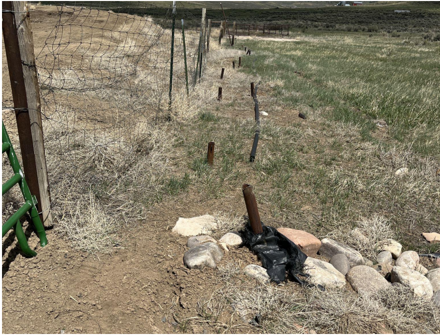
Photo 9. Photo taken from the east end of the pit facility outside of the fence, facing north. Photo illustrates anchor pipes, which have not been properly covered to prevent wildlife access, including birds and bats.
