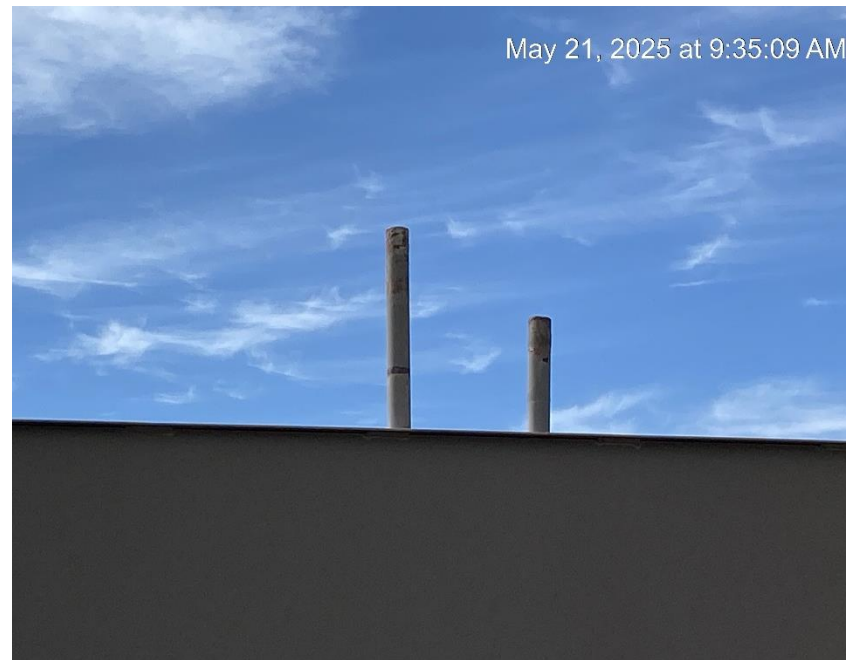
Unprotected relief vent risers
