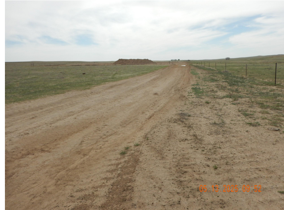
Photo 4. Photo taken from the western access road, facing East. See comments under Photo 1.
