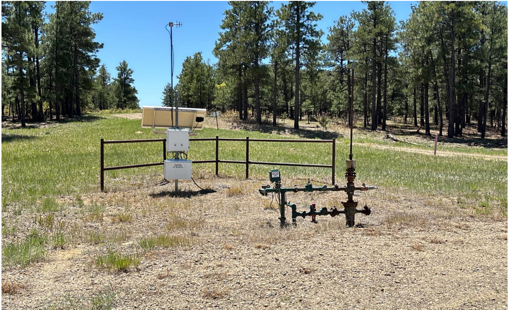
PHOTO 3: WELLHEAD AND EQUIPMENT.
