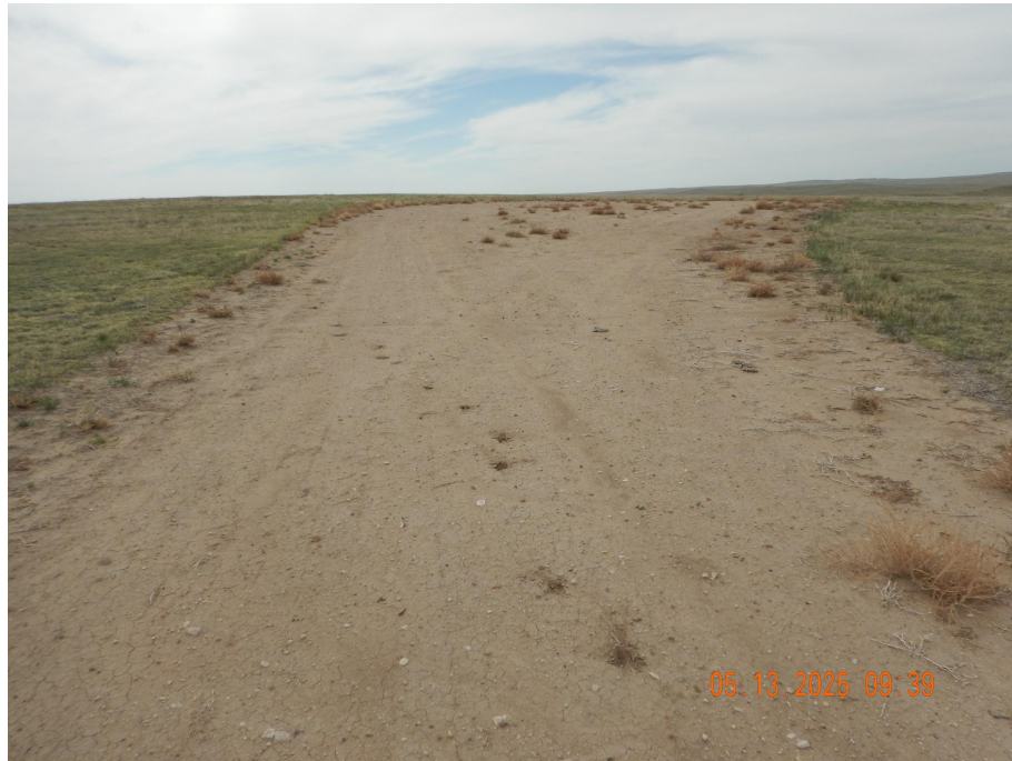
Photo 1. Photo taken from the northern location, facing Southeast. Photo illustrates the Operator has failed to perform final reclamation activities, which includes removing non-compliant topsoil and importing an approved topsoil source verified by ECMC Reclamation.
