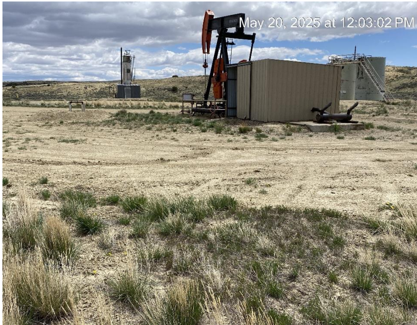
Location from Northwest corner
